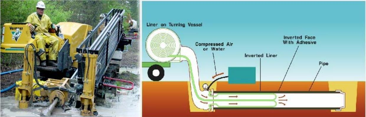
**Figure 3 – Trenchless technologies, such as a boring machine (left) and a hose liner (right), are technically and economically viable for various applications.**
